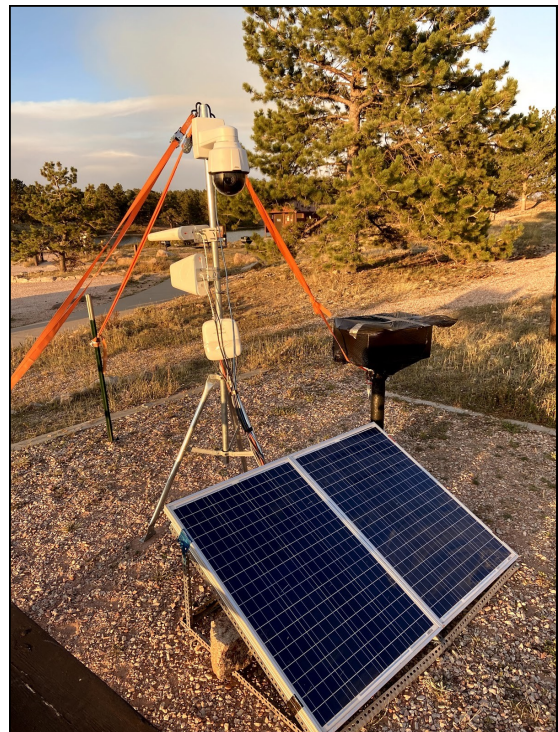
Figure 8— Camera and cellular data link in operation at Red Feather Lakes
