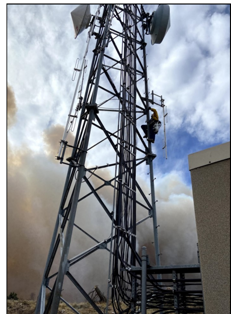
Figure 12— Larimer County radio technician installing camera at Horsetooth Mountain
